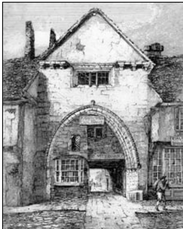
The Priory Gateway shortly before demolition to make way for the building of Priory Street.
